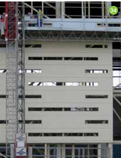
34 Kingspan KS1000FL panel installation at Doha airport
