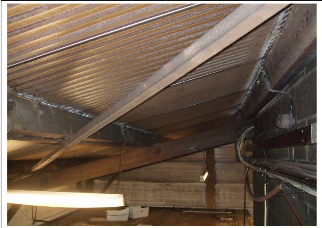
Figure 8 – view looking from the plant mezzanine level towards north wall
