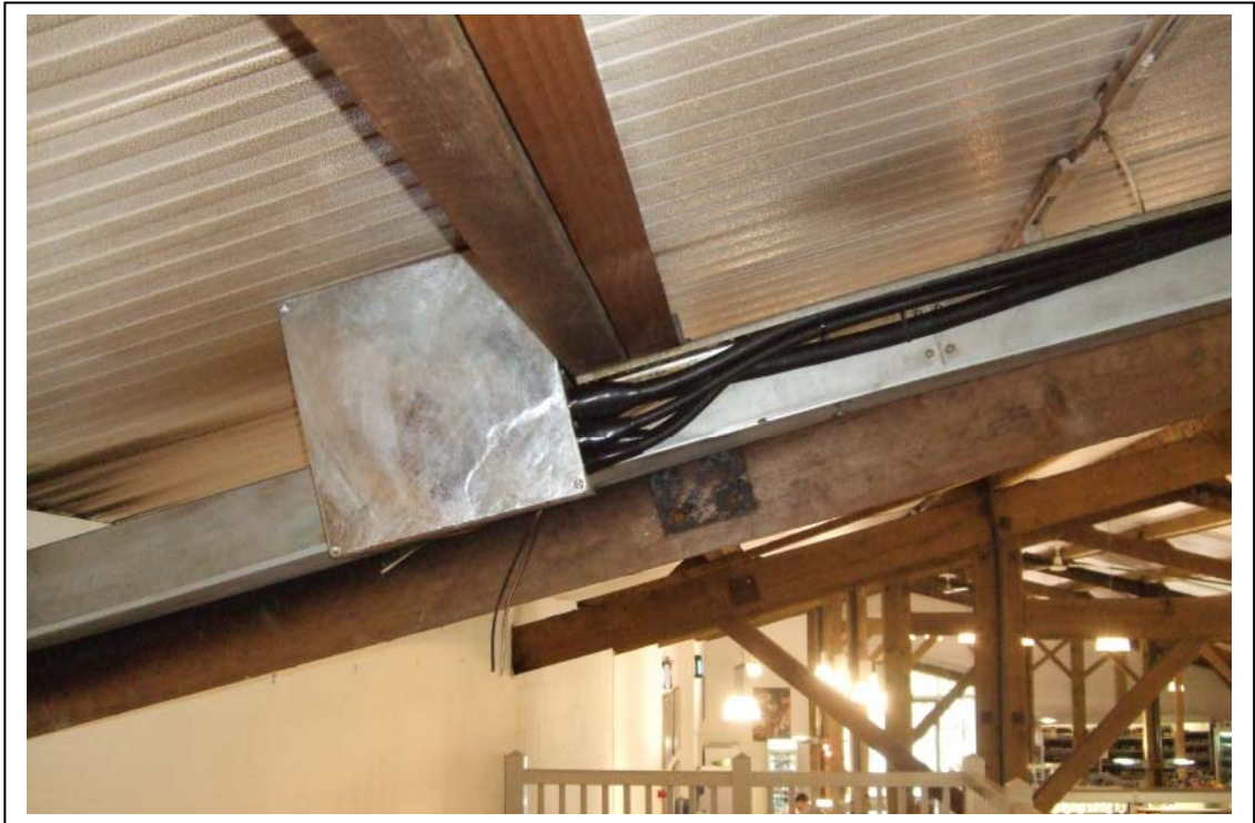
Figure10 – wall between mezzanine plant area and main sales space
