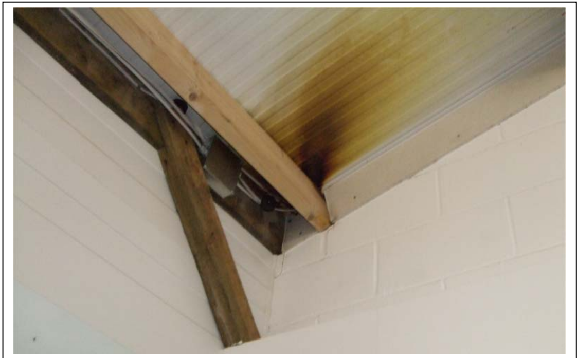
Figure11 - photograph of underside of roof in adjacent demise
